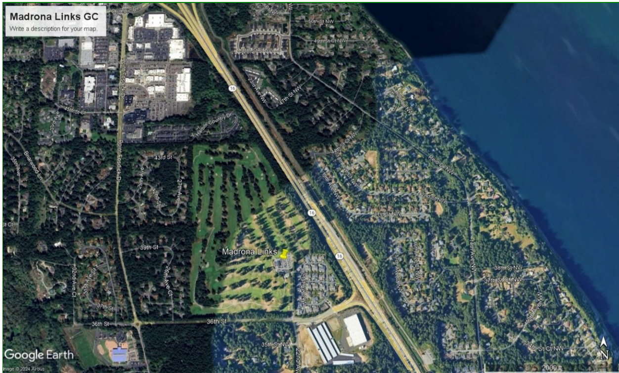
Google Earth image showing MLGC and direct surrounding elements, showing proximity to Highway 16 and local residential and commercial elements that provide some customer support for the golf course and clubhouse operation.
