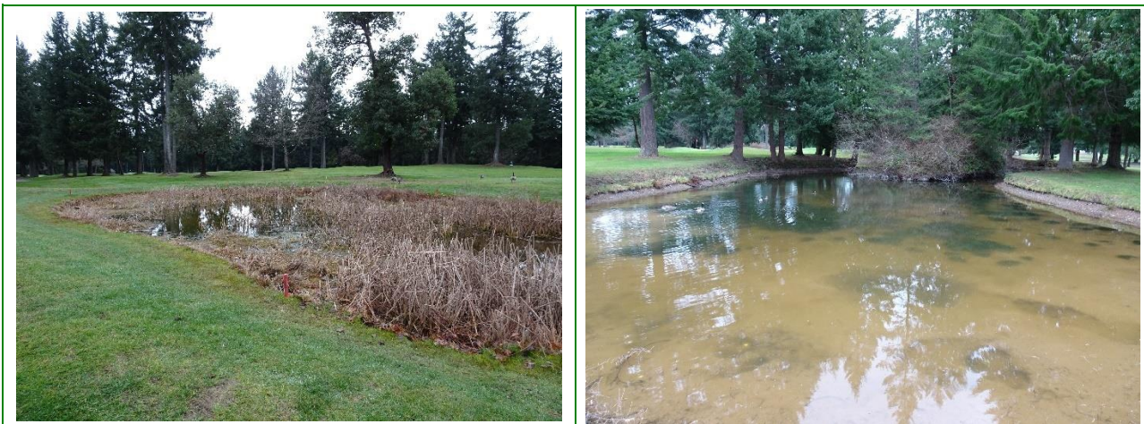
Images of ponds on MLGC. The algae buildup is unsightly, but the system is functioning, and the storage capacity is needed to appropriately distribute irrigation water to the golf course.
